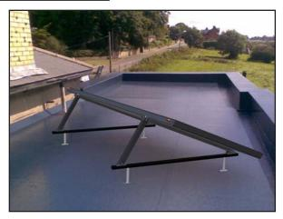
**Note:** In situations where the rack is to be mounted other than parallel to the roof line, cross bracing may be necessary. If you have any questions or feedback, please feel free to email us at sales&support@sunearthinc.com.
