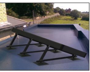
Note: In situations where the rack is to be mounted other than parallel to the roof line, cross bracing may be necessary. If you have any questions or feedback, please feel free to email us at sales&support@sunearthinc.com.
